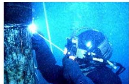
In wet welding MMA (manual metal arc welding) is used.
